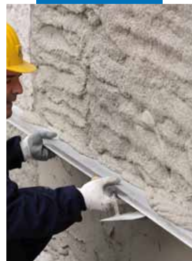
Levelling off the surface with a straight-edge PoroMap Intonaco Macchina
