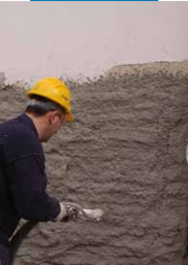
Application of PoroMap Intonaco Macchina
